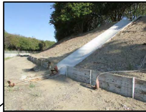
CONSTRUCT CULVERT TO REPLACE EXISTING DRAINAGE SWALE.
