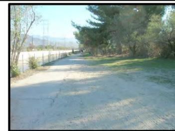
EXISTING ASPHALT MULTI-USE PATH. WIDEN PATH TO CHANNEL WALL AND OVERLAY WITH 2" FOR ASPHALT TO ACCOMMODATE A 12' CLASS 1 BIKE PATH.
