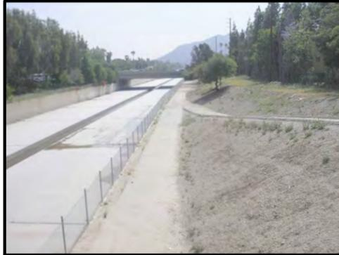
EXISTING 10' ASPHALT MAINTENANCE ROAD WITH VEHICLE ACCESS. EXISTING CHAIN LINK FENCING ALONG CHANNEL WALL. WIDEN PAVEMENT AND OVERLAY EXISTING PATH TO ACCOMMODATE 12' CLASS 1 BIKE PATH.
