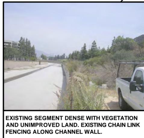
EXISTING SEGMENT DENSE WITH VEGETATION AND UNIMPROVED LAND. EXISTING CHAIN LINK FENCING ALONG CHANNEL WALL.
