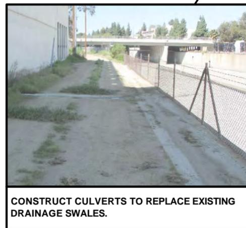
CONSTRUCT CULVERTS TO REPLACE EXISTING DRAINAGE SWALES.
